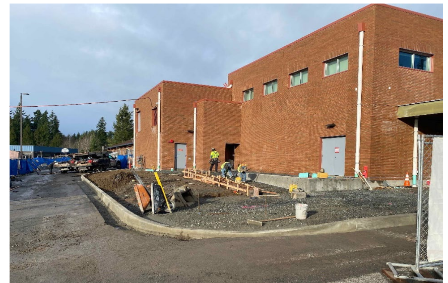
Canyon Creek Gym addition
